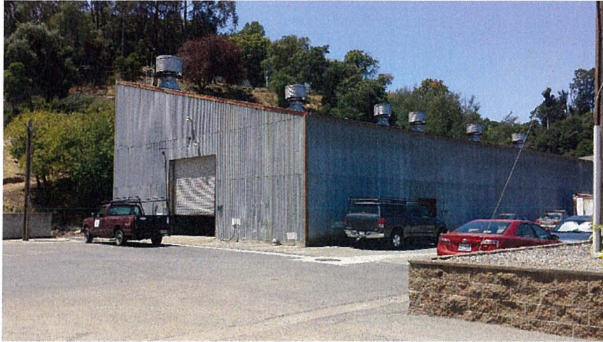
General outside view of Bldg. 86
