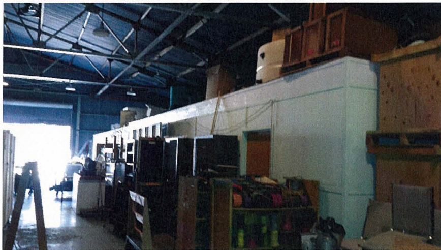
Storage on top of Office Area
